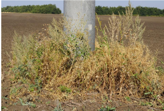
Fig. 4. The size of the spot overgrown with weeds.
